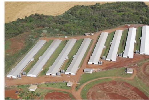
Poultry house heating
