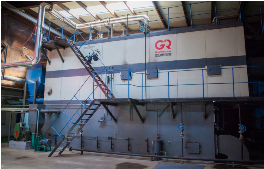
Supplying steam (2*10.5MW biomass boiler) to drug producer
