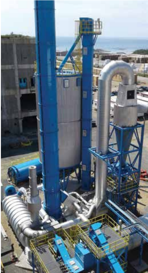
Ensyn's 10-million-gallons per year pyrolysis oil plant in Port Cartier, Quebec, Canada is the largest thermal conversion plant in the world.
