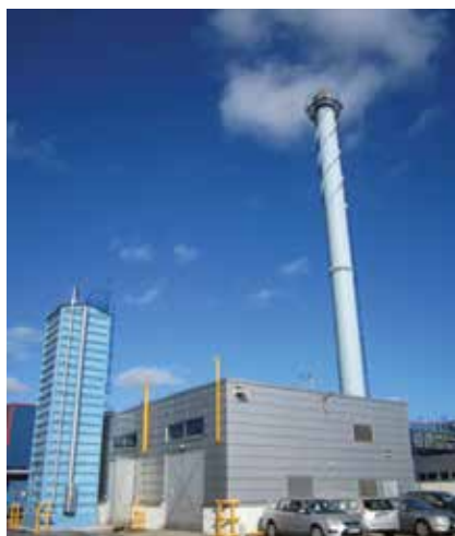
An Enerstena wood pellet boiler house for steam generation for an industrial company in Lithuania.
