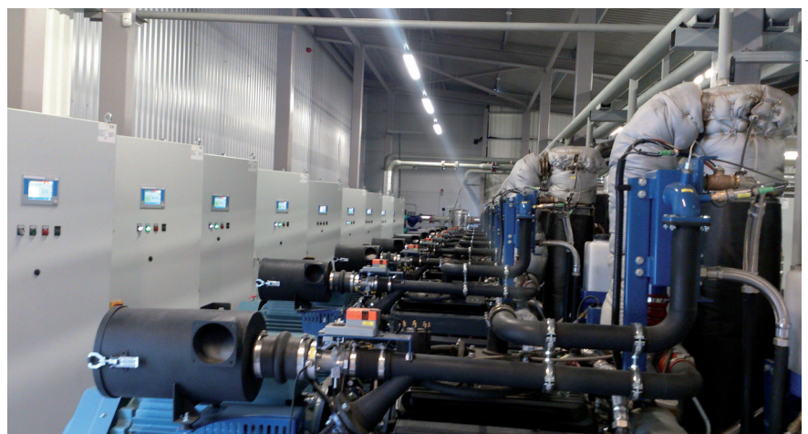
Figure 12. Woodchips cogeneration plant to produce electricity and heat. This plant includes 10 x 45 kW biomass gasifier & CHP installed in the city of Jaunjelgava, Latvia. Ten independent units generate 450 kW of electrical power and 1.08 MW of thermal power. The plants in Jaunjelgava provide a school, a kindergarten and several blocks of flats with heat at 2 ct/kWh. The electricity produced is fed into the national grid at 14 ct/kWh. The total investment was 4700 €/kW e . The charcoal which accumulates during gasification is collected in big bags and sold to Poland.
