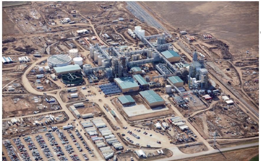
Figure 5: Abengoa advanced biofuels plant, Hugoton, Kansas, USA.
