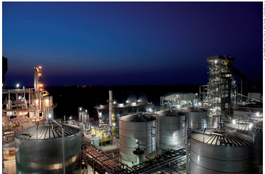
Figure 6: Novozymes/Beta Renewables advanced biofuels plant, Crescentino, Italy
